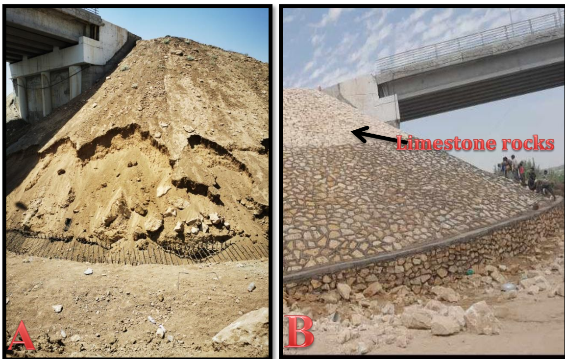
Fig. 1: Slope resulting from the construction of the newly built Al-Shohadaa Bridge on the Tigris River/Ninavah Governorate, (A) the condition of the slope before (stones riprap), (B) the condition of the slope after (stones riprap) with limestone rocks.
